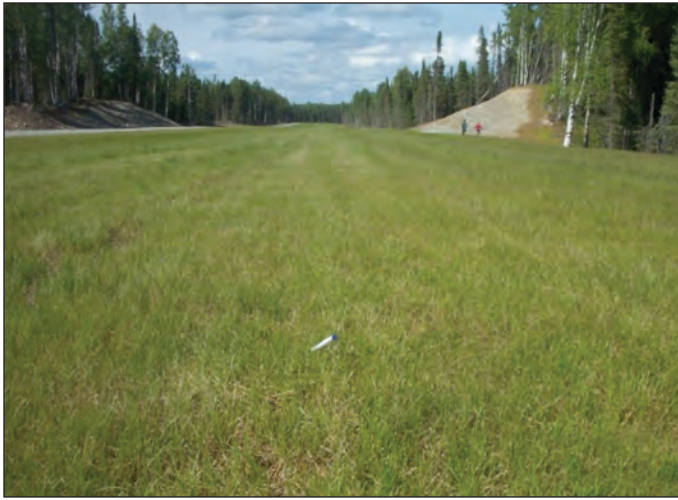
Figure 3. The Arctared red fescue grass planted on this runway has the potential to greatly reduce damage caused by rocks. The grass also reduces dust. Photo by Jud Scott
