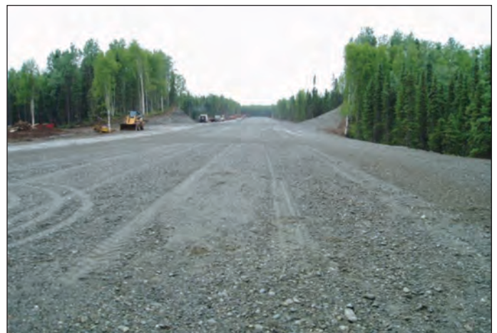
Figure 2. Newly created gravel runway in August 2008. The unconsolidated rocks represent a safety and financial hazard for airplanes and their owners.
