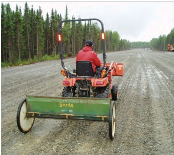
Figure 5. A tractor with a drop spreader was used to plant this runway. An ATV with a broadcast spreader will also work. Notice that planting took place during a light rain, which helps with germination. Photo by Tim Evers
