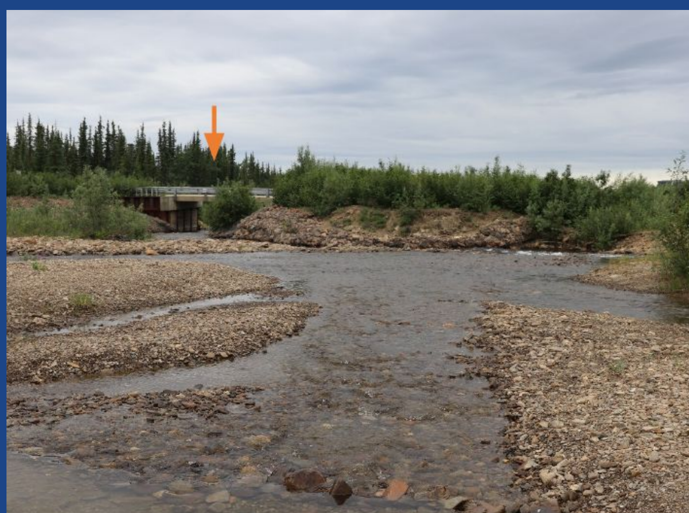
Figure 1: Nome Creek prior to restoration. Reach is just upstream of the U.S. Creek Road bridge.
