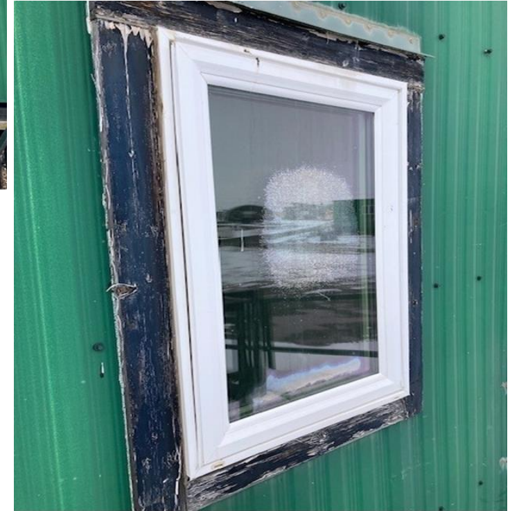
Winter Lab window with broken seal.
