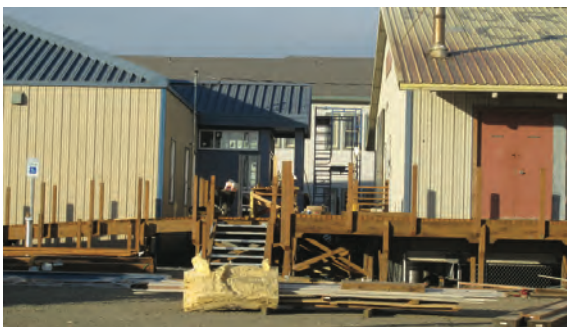
The main building (left) and library (right) were moved onto new pilings and are now just steps apart across a new deck area (photo taken during renovation)
