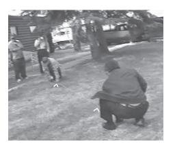
Fig. 5.8: Rechecking the diagonal distance.
