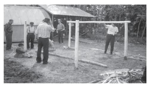
Putting in the posts and beams for the fish rack.
