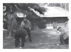
Fig. 5.6: Elders use a rope to determine the width. Arrows indicate the corners of the future fish rack
