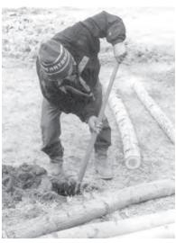
Fig. 5.9: Digging the holes for the posts
