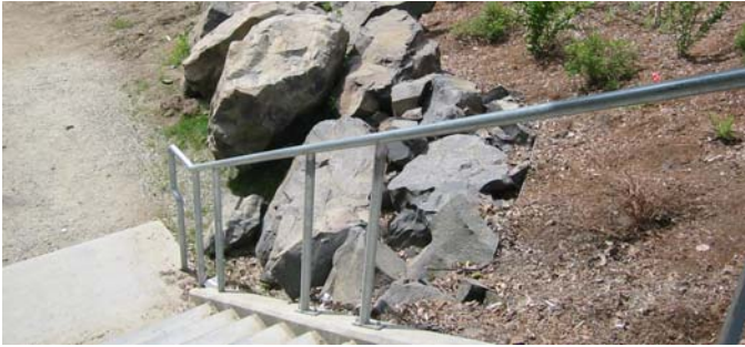
Boulders installed at the base of the slope and groundcover will reduce erosion.
