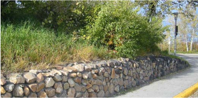
Boulders installed at the base of the slope and groundcover will reduce erosion.
