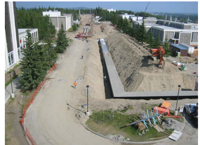
Construction of the Utilidor in the West Ridge, Summer 2003.
