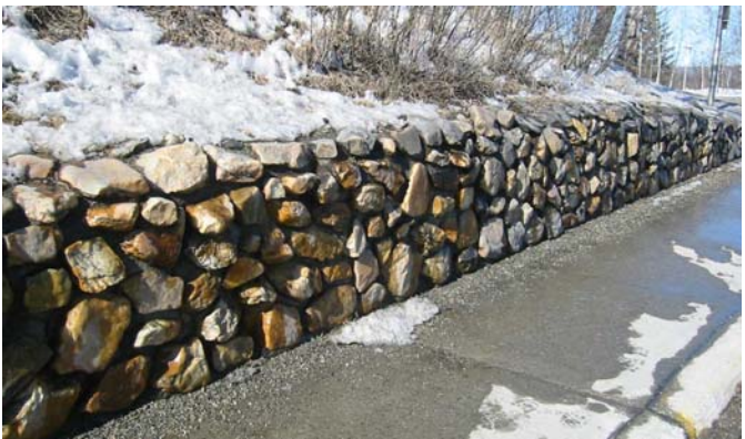
The stone retaining wall along North Chandalar is beautiful, but drainage should be redirected away from the sidewalk.
