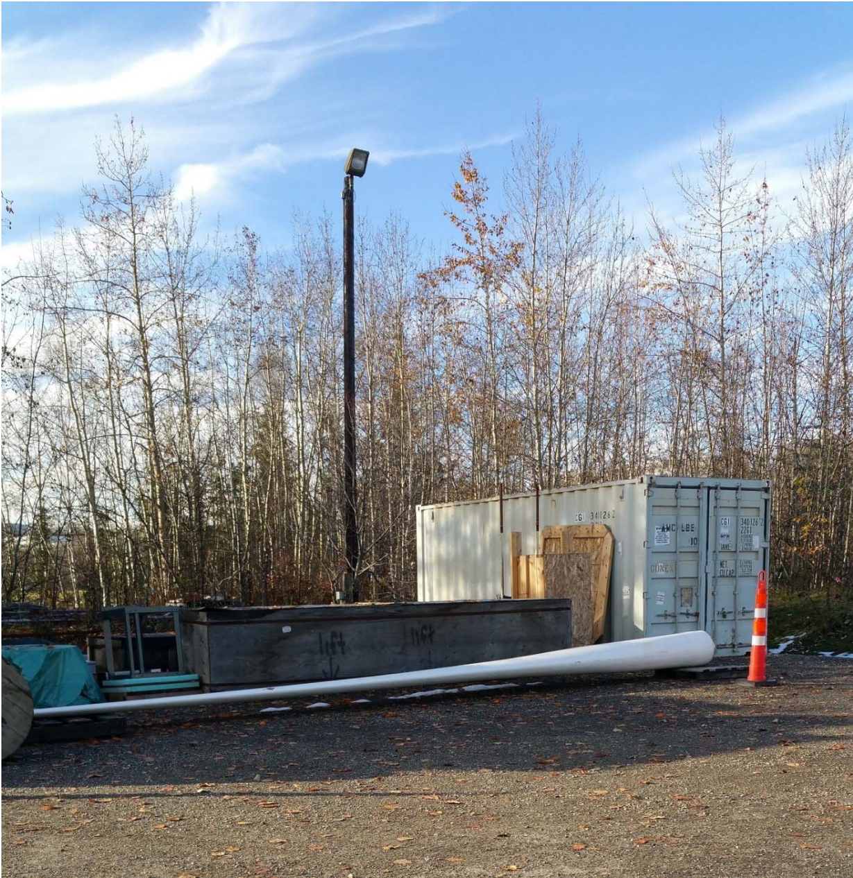
Connex and Storage at Energy Testing Module and Switch Gear Building
