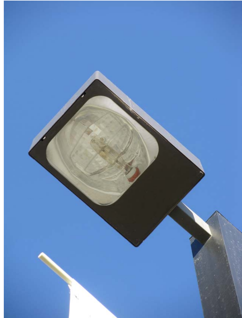
Typical "Shoebox" luminaire utilized in parking lots
