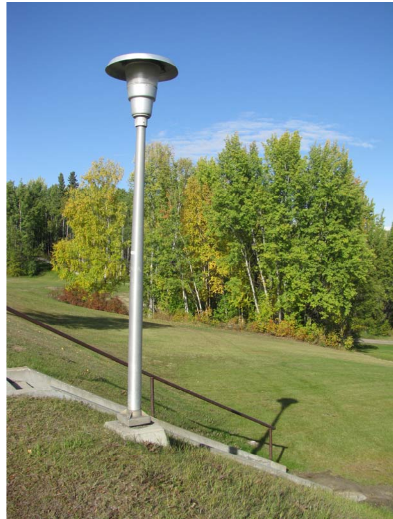
Typical “China Hat” luminaire utilized on campus walkways
