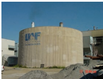
1.5 million gallon storage tank
