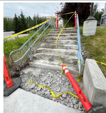
Concrete Repairs: Alcan Construction is repairing the concrete stairs at the 100 Building in the Cutler Apartment Complex. Years of winter maintenance caused the stair edges to deteriorate. This project, along with repairs to a stairway on the east side of the Patty Center walking deck, is scheduled for completion by August 15. photo by N. Platt
