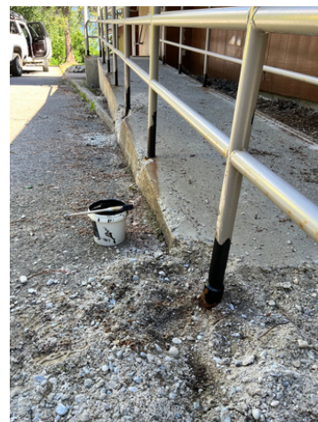
Chancellor's House Improvements: Repairs are underway at the Chancellor's House. The rust on the wheelchair ramp handrails has been treated, and since this photo was taken, James and Connor from the Carpentry Shop have completed concrete repairs. Upcoming work includes touch-up painting of the handrails, a kitchen update, and landscaping improvements. photo by N. Platt
