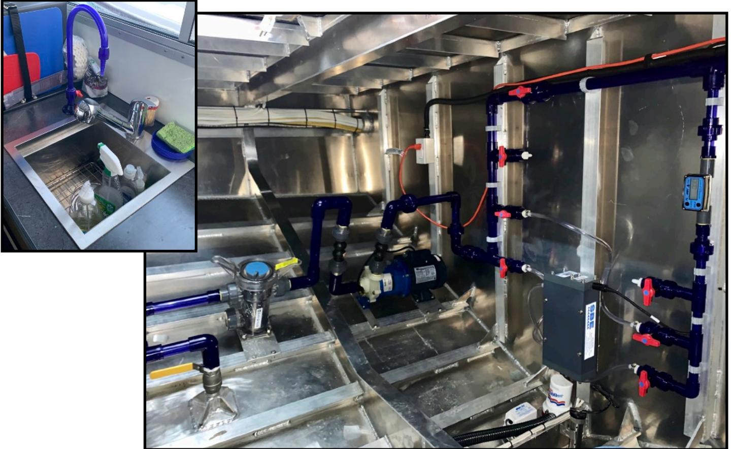
Spears Low-Extractable High-Purity PVC System was selected for all piping and fittings. This material is specially developed for ultra-pure water systems used in laboratories and hospitals. It is a non-contaminating material with exceptionally smooth surface characteristics, low TOC & chemical extraction, and fast particle rinse-up.
