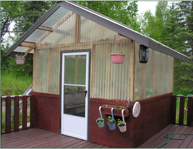
The gable style provides more headspace and room for growing plants than the A-frame or Gothic style.
