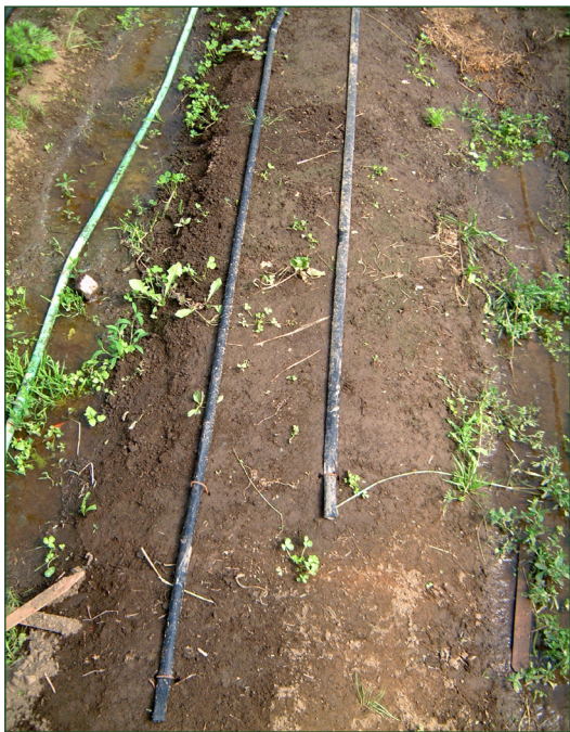
A greenhouse drip system uses water efficiently.
