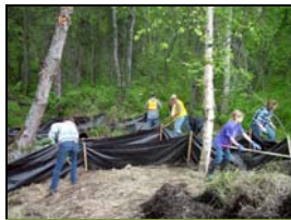
Mulch applied as erosion control during a restoration project. Photo: Wasilla SWCD
