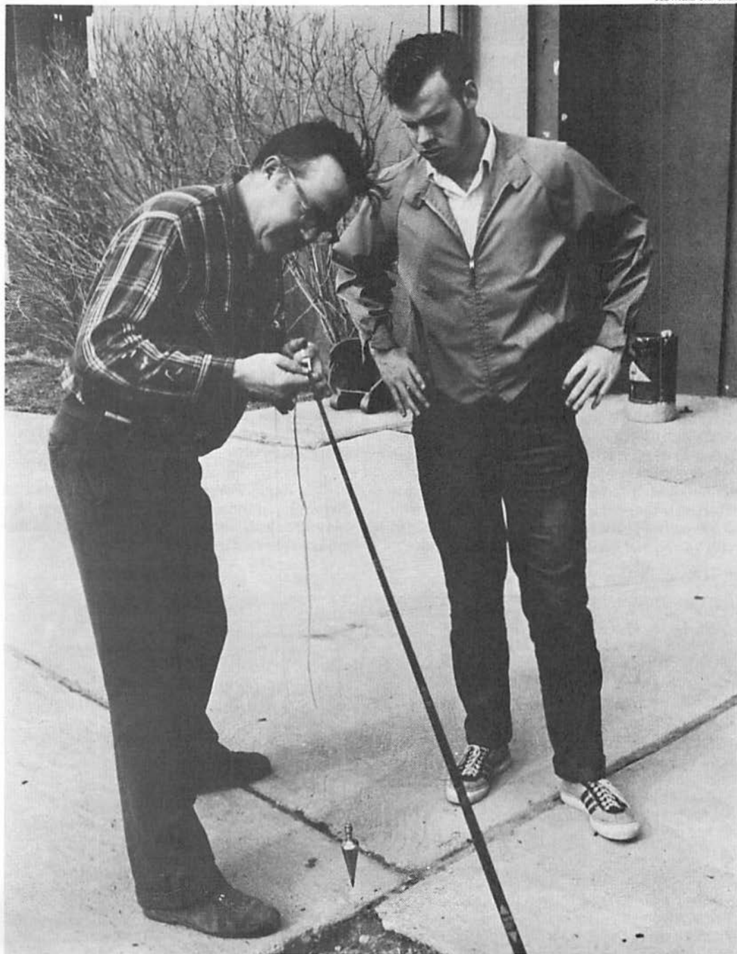
Students in a surveying course practice correct chaining technique.
