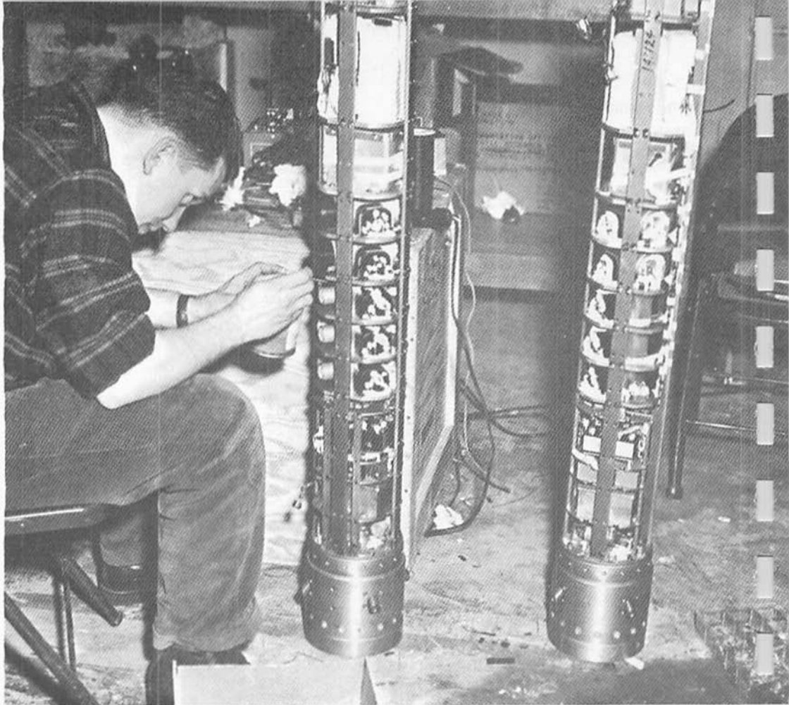
Studies of the aurora borealis are a key part of the research program of the Geophysical Institute. Here, a scientist adjusts a rocket assembly used in conducting upper atmosphere aurora studies.
