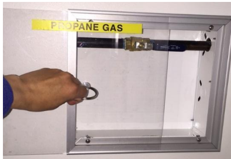
Figure 3. Removal of Plexiglass plate covering valve
