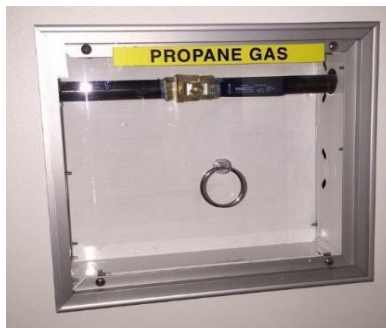
Figure 2. Propane gas shut-off valve
