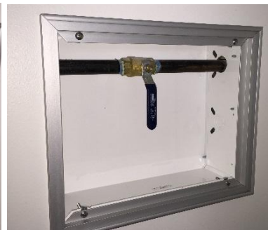
Figure 4. Valve handle in "off" position
