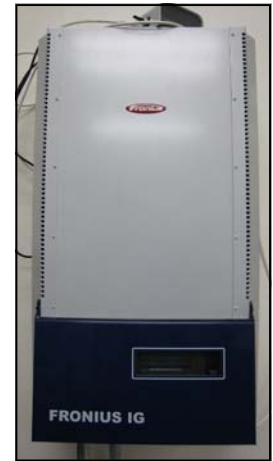
This gray box is a fancy electrical box, called an inverter that connects UAF BBC’s solar panels to the electric grid.
