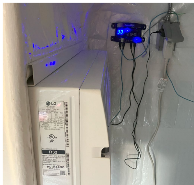
Figure 3 Images from the oyster cold storage unit, including shelving and “cool-bot” controlled air conditioning.
