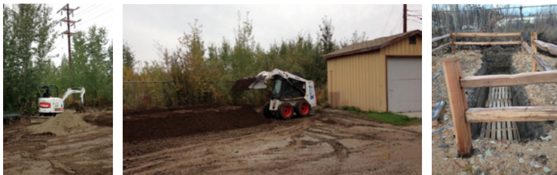
Figure STEAM 10. Facilities Services creates the University Park Forest Education Outreach Center on University Avenue near campus. Left: excavating the trench. Center: building transplant beds. Right: the finished 18' x 4' x 4' trench, ready to receive overwintering tree seedlings and insulated cover.
