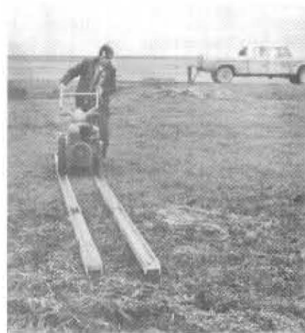
Agronomists lay first "tundra railroad" on North Slope to transport a rototiller across hummocky terrain.
