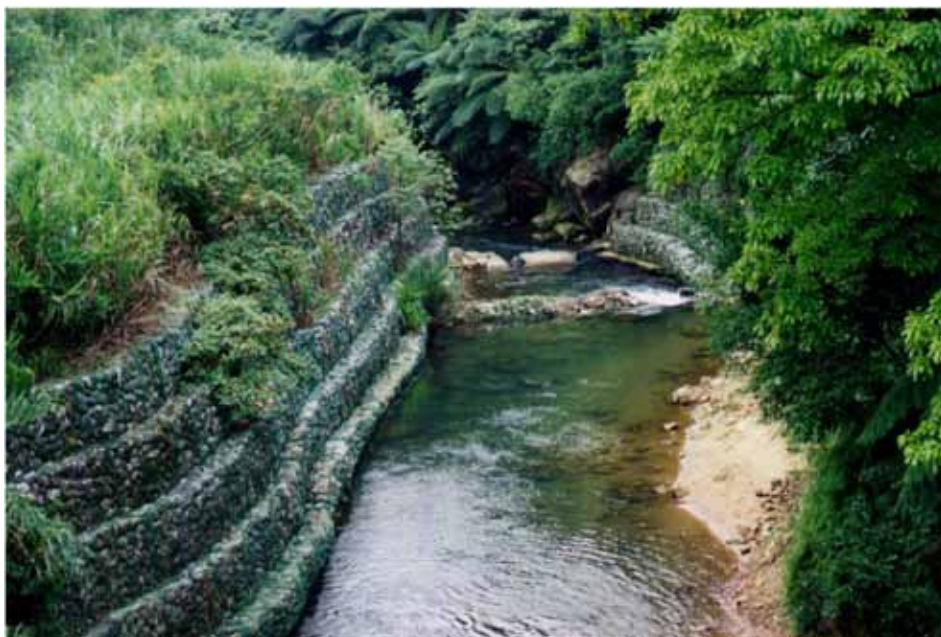
Riverbank stabilized with rock cages.
