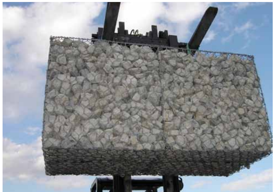
Rock cage: Wire cage filled with crushed rocks or gravel being lowered onto the river bed.
