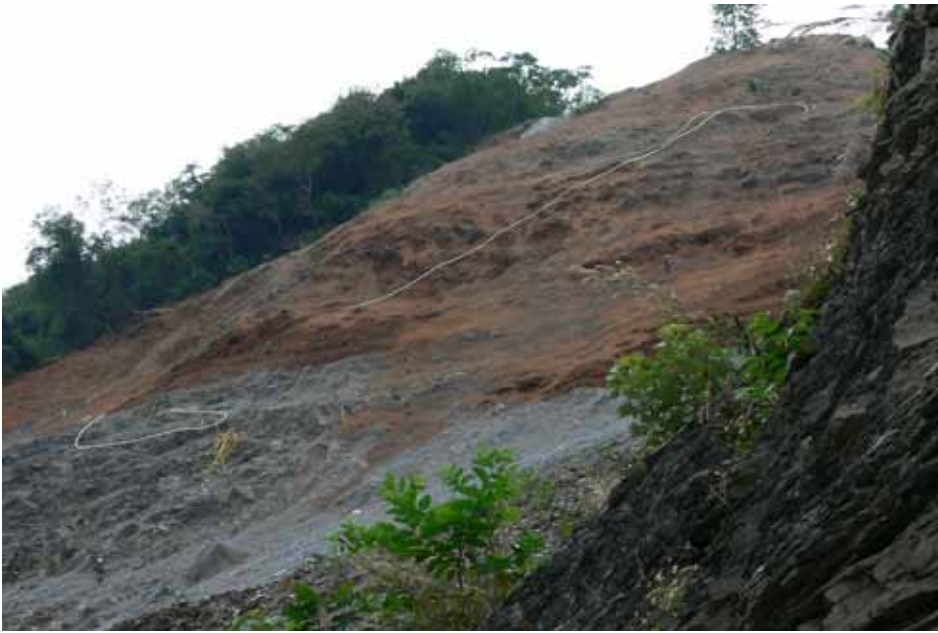
Landscape experts and construction workers lay nylon nets over a steep slope where the soil and vegetation were stripped by Typhoon Morakot. The nets are anchored and vegetation replanted.
