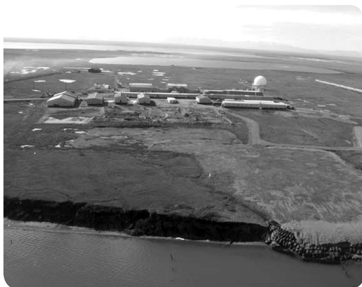
Sandbags shore up the bluff at the Flaxman Island site of an abandoned Dew Line facility that is east of Deadhorse, between Deadhorse and Barter Island.
