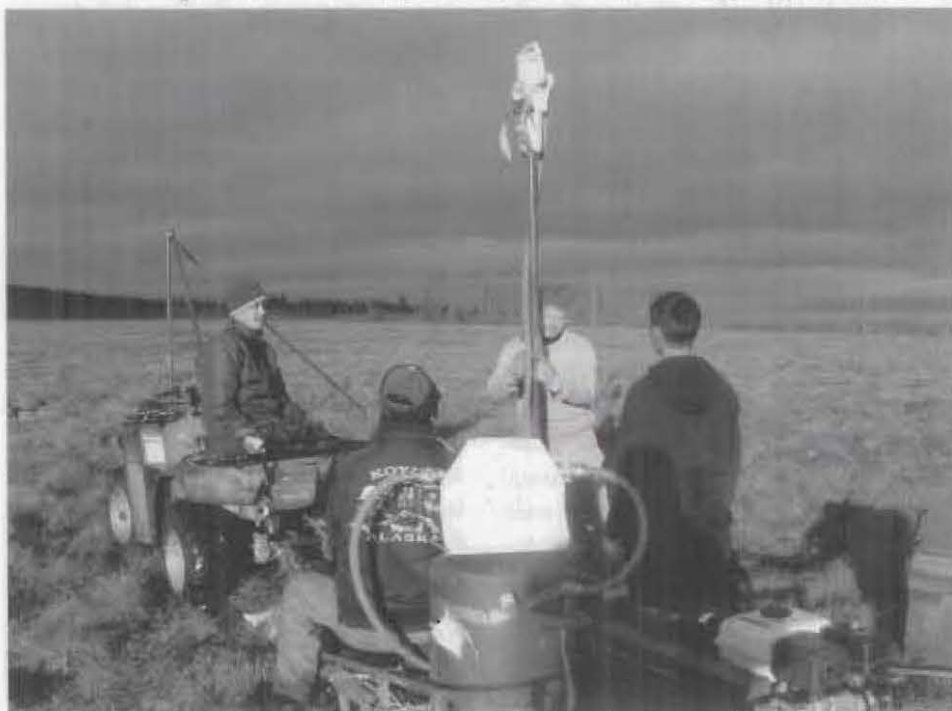
Merlin Henry (center, facing away from camera), two of his nephews, and Greg Finstad (center, facing toward camera), who is using a pneumatic post pounder in 2005 to construct an enclosure for Henry's reindeer.
