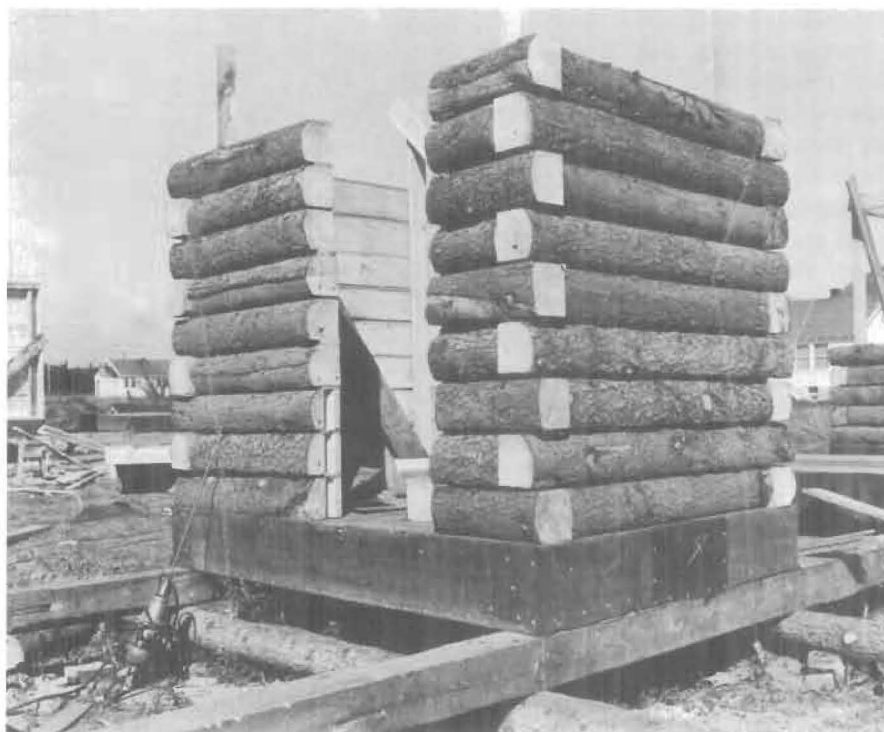
Photo shows walls being constructed on spruce log experimental cabin
