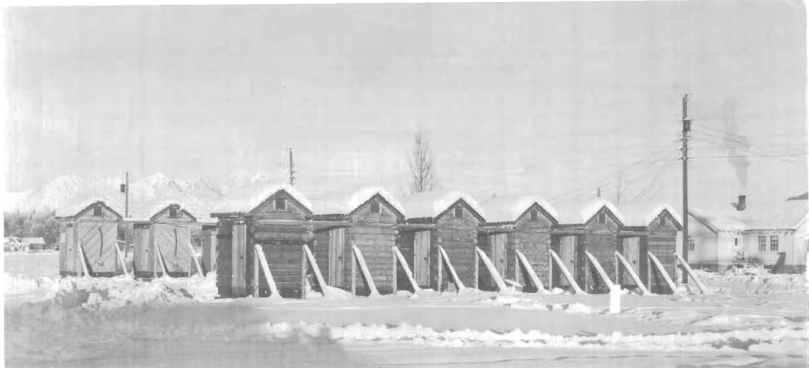
Cold roof design of experimental cabins shows no icicles and a heavy snow cover. Several insulating materials were tested.
