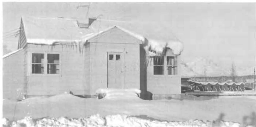
Iceicles hang from uninsulated roof of home in Palmer. Branton's cabins at right.
