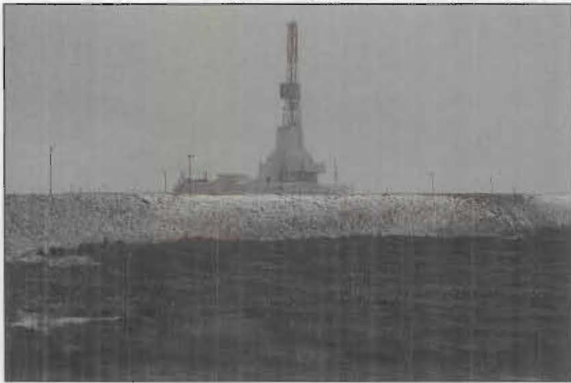
A drilling rig operates on a gravel pad near the Kuparuk River, just west of the Prudhoe Bay Oil Field (September 22, 1989). Observe the thickness of gravel used to provide a stable surface for operating heavy equipment in this region of continuous permafrost.
