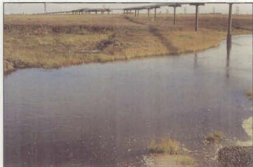
This pipeline carries crude oil from the Lisburne Oil Field. The pipeline crosses the Little Putuligayuk River en route from the Lisburne Production Center, operated by ARCO Alaska, Inc., to Pump Station No. 1 of the Trans Alaska Pipeline, operated by Alyeska Pipeline Service Co. Notice the clearance under the pipeline provided for caribou and the absence of a work pad. This pipeline was constructed in the winter of 1985-86 and represents technology of the mid-1980s. (photo taken September 1, 1989)
