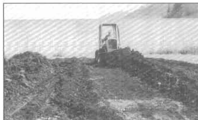
Figure 2. A bulldozer worked and reworked the oil sludge and topsoil to produce the oil sludge/soil mix.
