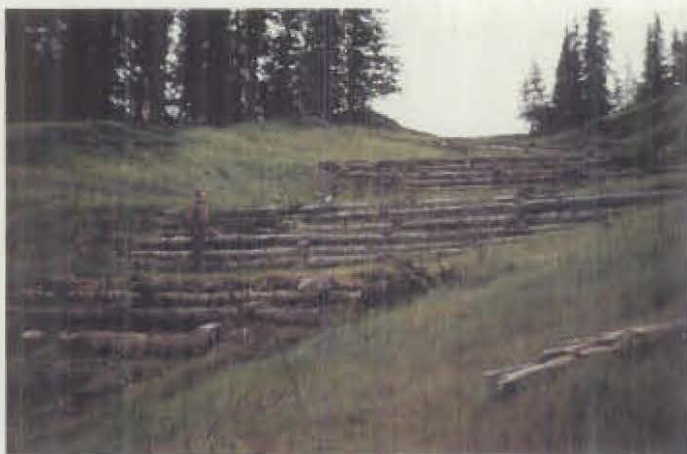
Early conservation practices often utilized available materials, as shown by this erosion-control structure made out of logs.
