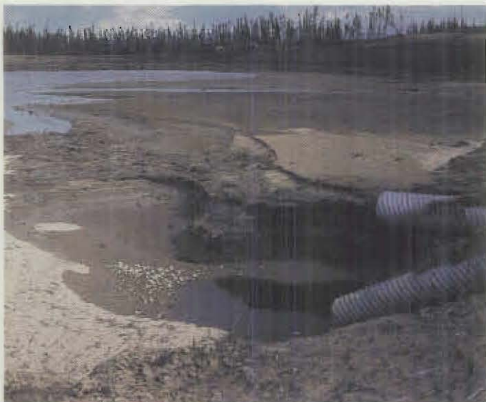
The force of water erosion can also cause damage to such man-made structures as culverts and roadbeds.
