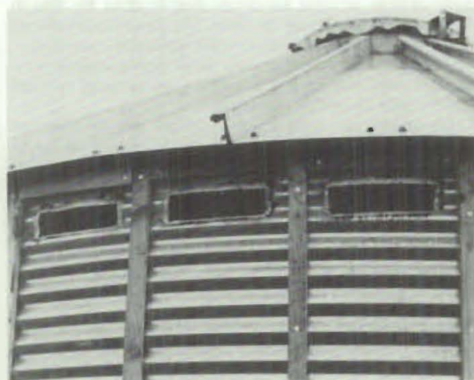
Figure 3. Holes were cut in the bin wall at the top of the air passages to admit warmed air to the bin.
