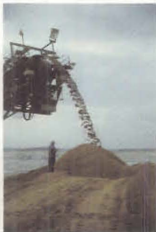
Coarse-textured materials are used to construct roadways among reclaimed fields of the surface coal mines near this West German town. That practice not only provides better roads, but also saves valuable loam soils for crop production.
