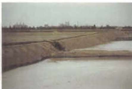
Slurries of loam are pumped into dyked areas during the reclamation of West German coal mine spoils.
