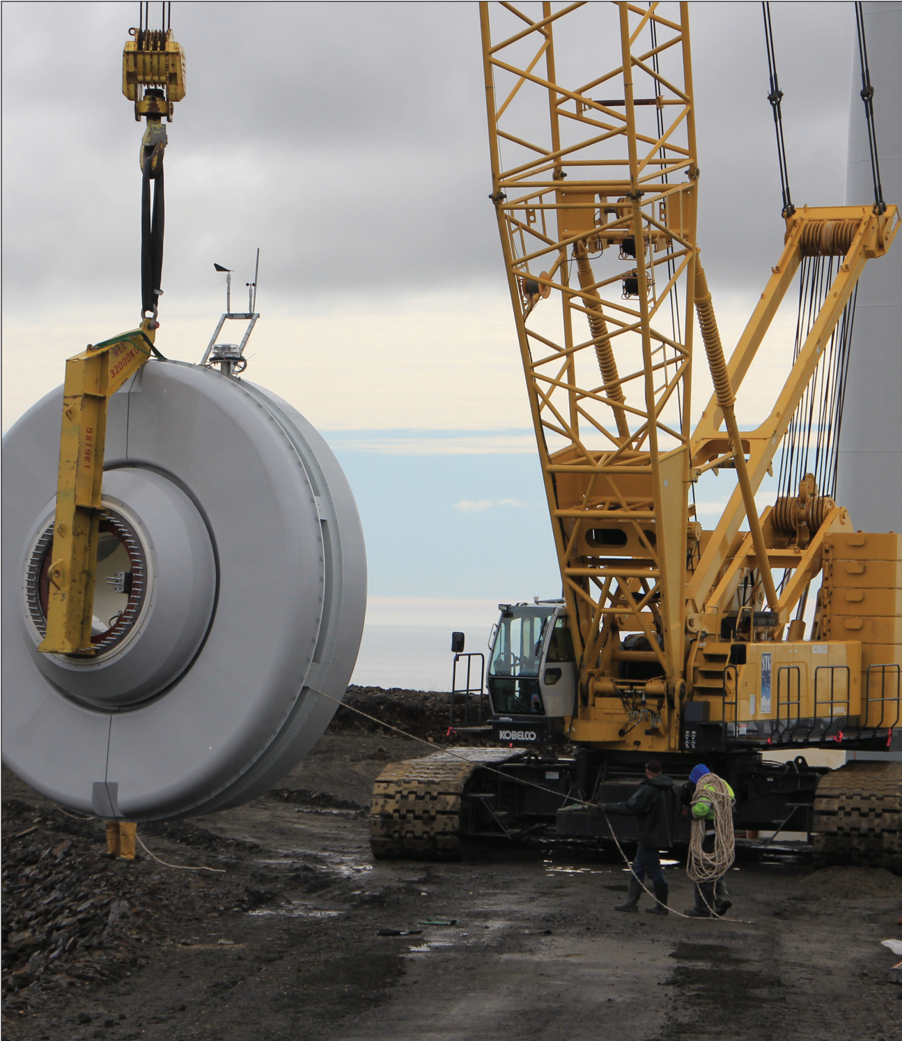
Nacelle of a 900 kW EWT direct drive wind turbine being lifted into position during construction of the second phase of the Banner Wind Peak Farm near Nome. Photo by Gwen Holdmann, ACEP.
