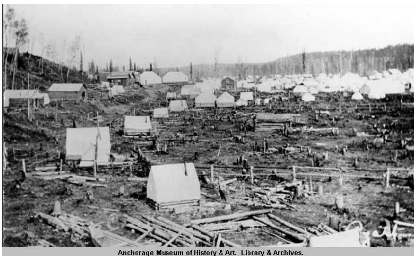
Figure 2: Clearing Land to Construct a Tent City on Ship Creek, Early Summer, 1915.
