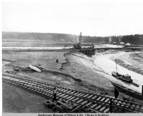
Figure 8: Railroad Bridge Construction, Ship Creek, 1915.
