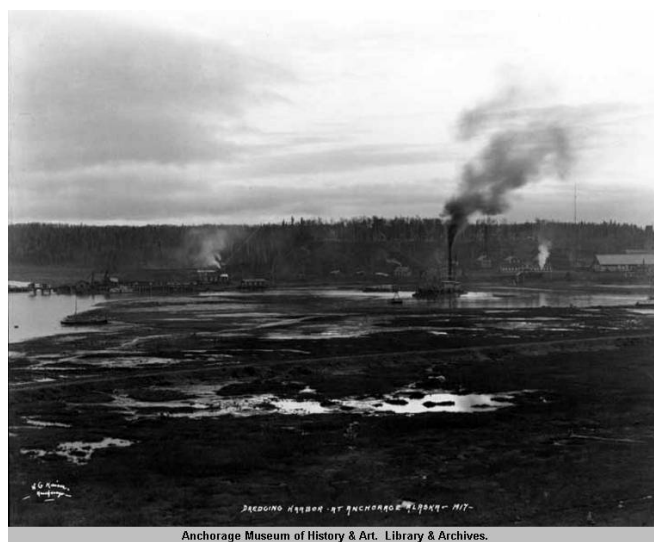
Figure 6: Alaska Engineering Commission Dredges Ship Creek, October 7, 1917.
