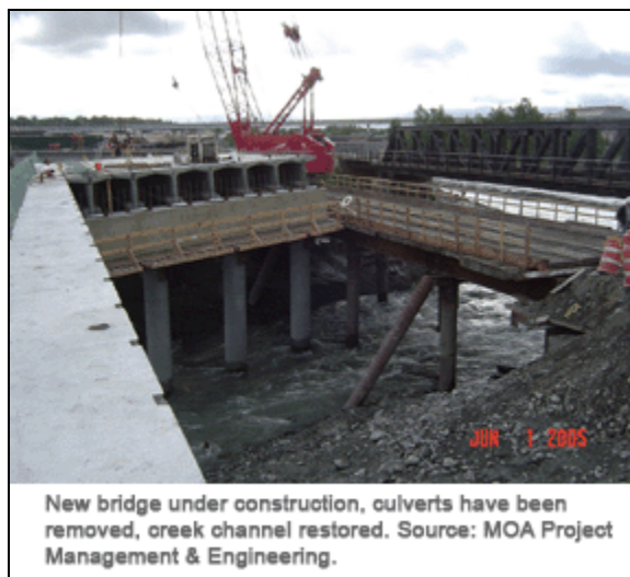
Figure 21: Construction of Bridge over Ship Creek, 2005.
