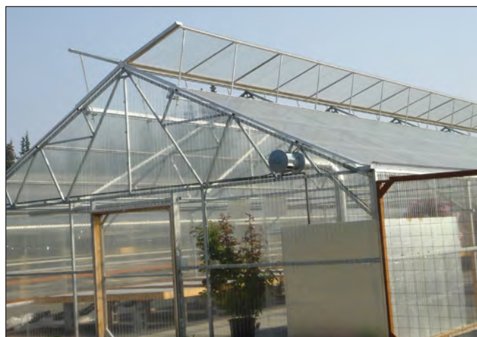
Picture 2: Roof ridge vents are shown at Trinity Greenhouse in Kenai.
