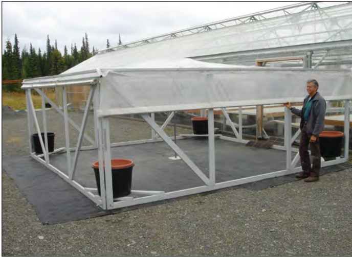
Picture 3: The drop-down wall design provides inexpensive but effective ventilation.
