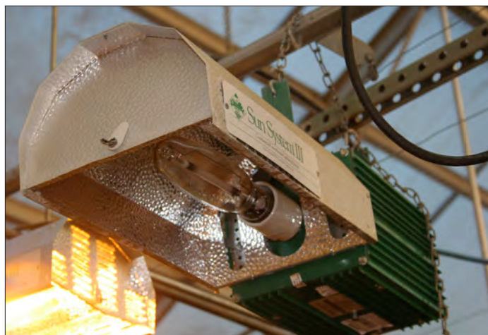
Picture 6. HID lamp with bulb, reflector and ballast/capacitor
