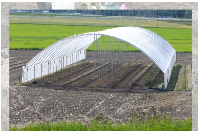
We decided to use the 7 oz. woven mesh plastic as opposed to the 6 mill plastic due to concerns for strength and durability over the winters.
