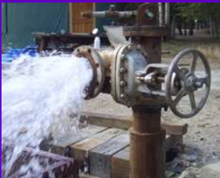
Geothermal Wells Provide Hot Water (~165F)
