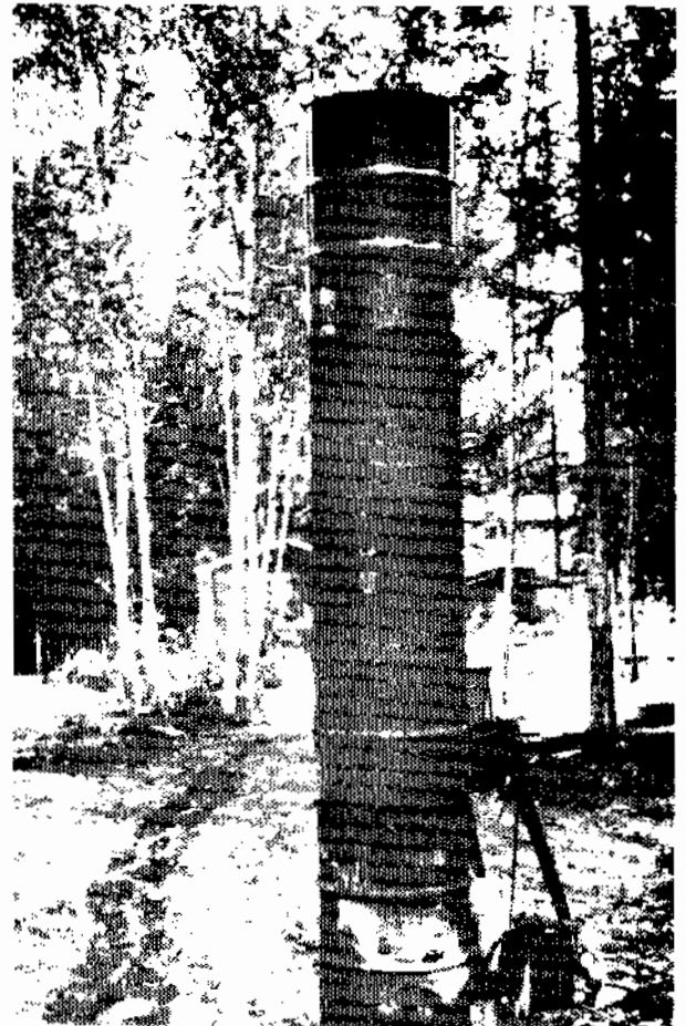
Burner # 2 in operation. Notice absence of smoke at top of burner.
