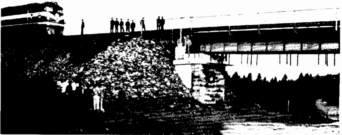
Steel plate girder bridge on the Yalin Line between Yakeshi and Mangui. Permafrost has been degrading under the riverbed, and there are access tubes in the river and the abutment that are used to measure temperatures.
