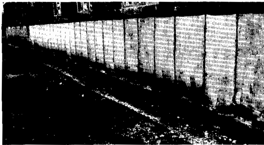
The foundation for a large apartment building to house railroad workers in Mangui. The structure, built on permafrost, was elevated approximately 1 meter above the ground surface. The holes near ground level provide ventilation to the space under the building. (Larry Sweet photo.)
