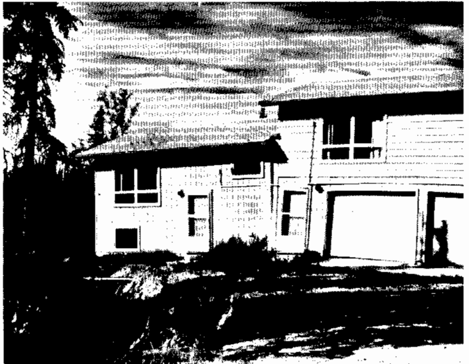
FIGURE 4. Sometimes "on-grade" construction can be disappointing.
