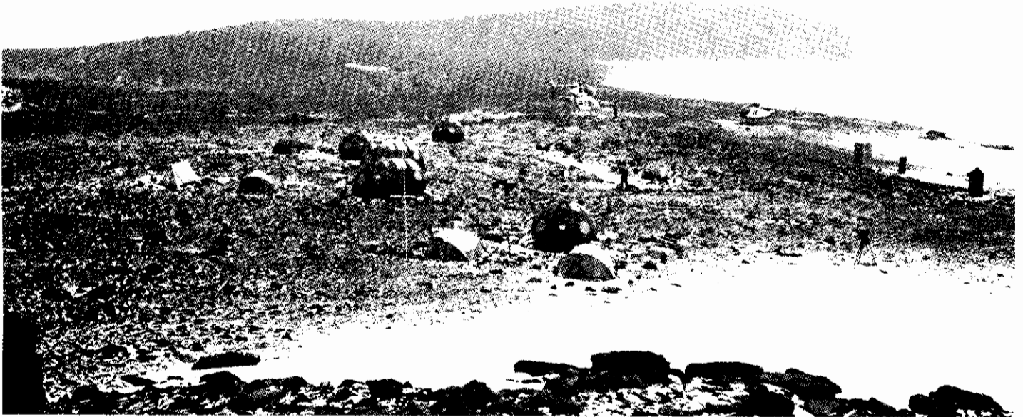
Edgeworth-David Summer Base, Bunger Hills, Antarctica, established in February 1986. The base comprises three basic Igloos (radio-meteorology, photographic darkroom, and living quarters) and two extended Igloos (mess and living quarters). Summer operations involve about 25 people. The shelters remain over winter. (Photographs and figures courtesy of AAD; photographs by Rowan Butler.)
