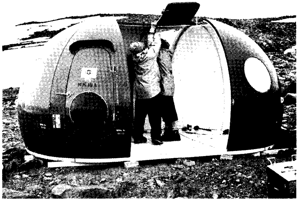
Extending a basic Igloo shelter by the addition of floor and side panels which had been airlifted inside the Igloo.
