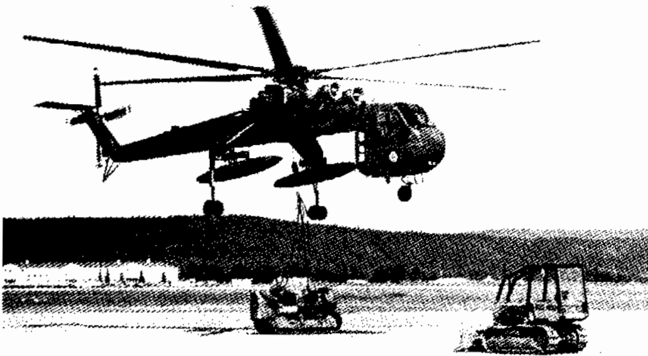
An Alaskan National Guard CH-54A Sky Crane lifts a bulldozer at Fort Wainwright for fire fighting in interior Alaska. Airlifting heavy equipment in Alaska requires special care to reduce buildup of electrostatic charge. (Photos courtesy of the U.S. Army.)
