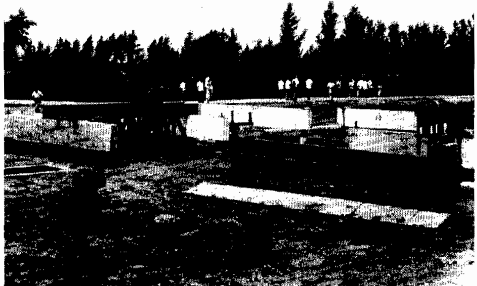
Figure 4. Field installation to measure frost heave on piles and footings. Field station of the Heilongjiang Provincial Scientific Research Institute of Water Conservancy, 19 km west of Harbin, China, July 19, 1984. (T. L. Péwé photo no. 4807.)
